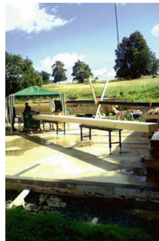
This is the photo that Per-Arne took with his cellphone, showing the planing of a 12 metre long beam with the measurements 8" x 12".
