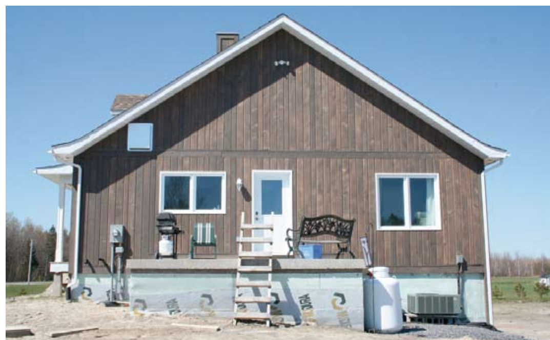
The White Pine siding is produced with the 4-sided PH 260 planer moulder.
