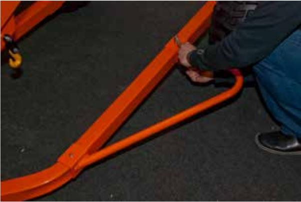
13. Fit the wheel guards on each side of the frame, as seen in the picture. Use **four M8x80** including **M8 lock nuts** with **M8 washers** on the side where the nuts are.
